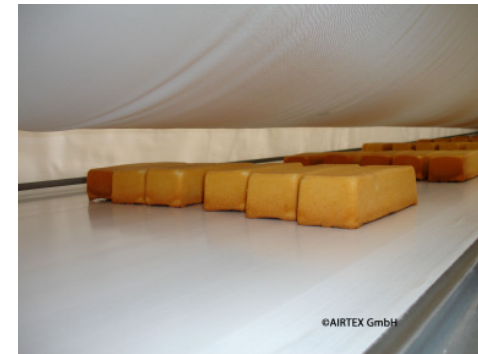
Textile ventilation ductwork Airtex Bioactive for cooling of bakery products in a wholesale Bakery. Photo: Airtex GmbH Textiler Luftkanal Airtex Bioactive zur Kühlung von Backgut in einer Großbäckerei Photo: Airtex GmbH
